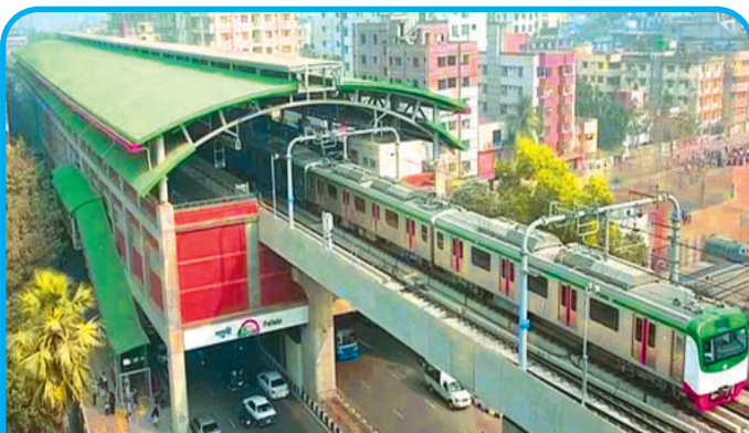
Dhaka Metro Rail: Project CP-03-04 & CP-06
