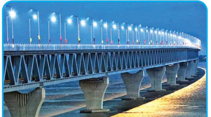
Padma Bridge Roadway Lighting
