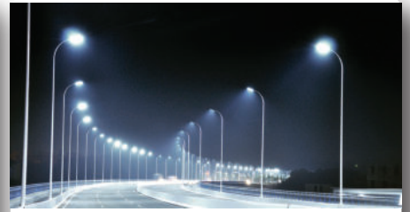
High Mast Lighting
